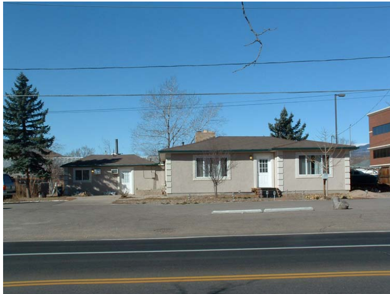
Figure 8. 2675 Youngfield Street (5JF4324), Looking West
