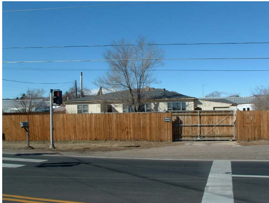
Figure 7. 2665 Youngfield Street (5JF4323), Looking West
