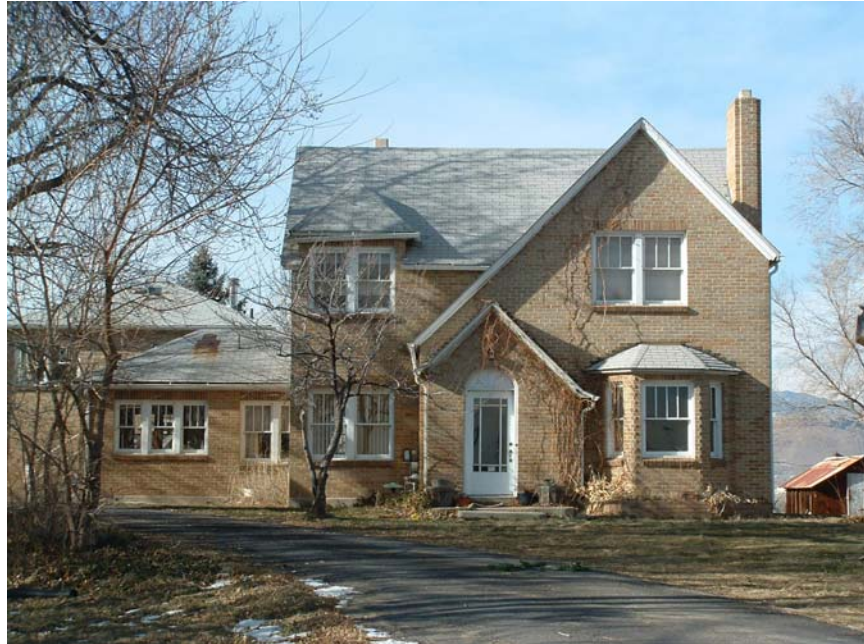
Figure 5. Salter Farmhouse, 3803 Youngfield Service Road (5JF3803), Looking West
