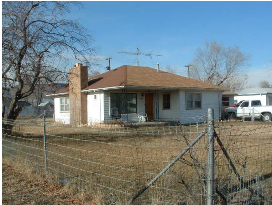
Figure 16. 4405 Holman Street (5JF4333), Looking Northwest
