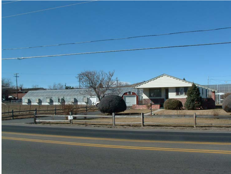
Figure 6. Novacek’s Carnation Nursery, 2635 Youngfield Street (5JF4322), Looking Southwest
